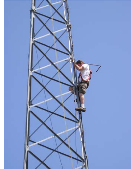
Barry McElroy placing BreadCrumb® on tower
